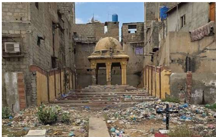
The Lady Phyllis Louise Lawrence's tomb, encroached upon by residential buildings from three sides, and covered with trash.
